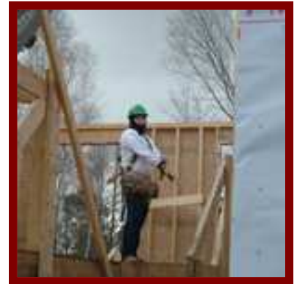
Student House Building Project
