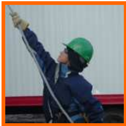
Student House Building Project
